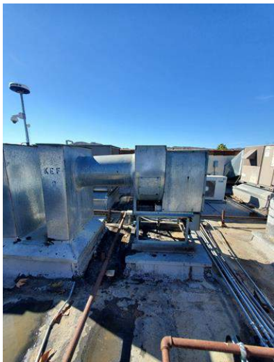
Description: York 8.5 Ton Gas/Electric Unit w/vfd M&M Invoice #062213, 8/11/20
