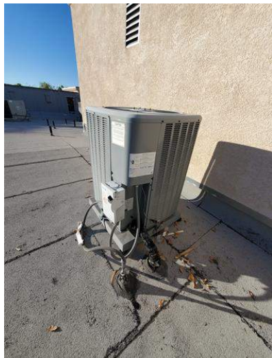
Description: July 2023, M&M, Replace Unit #28, $11,150.
